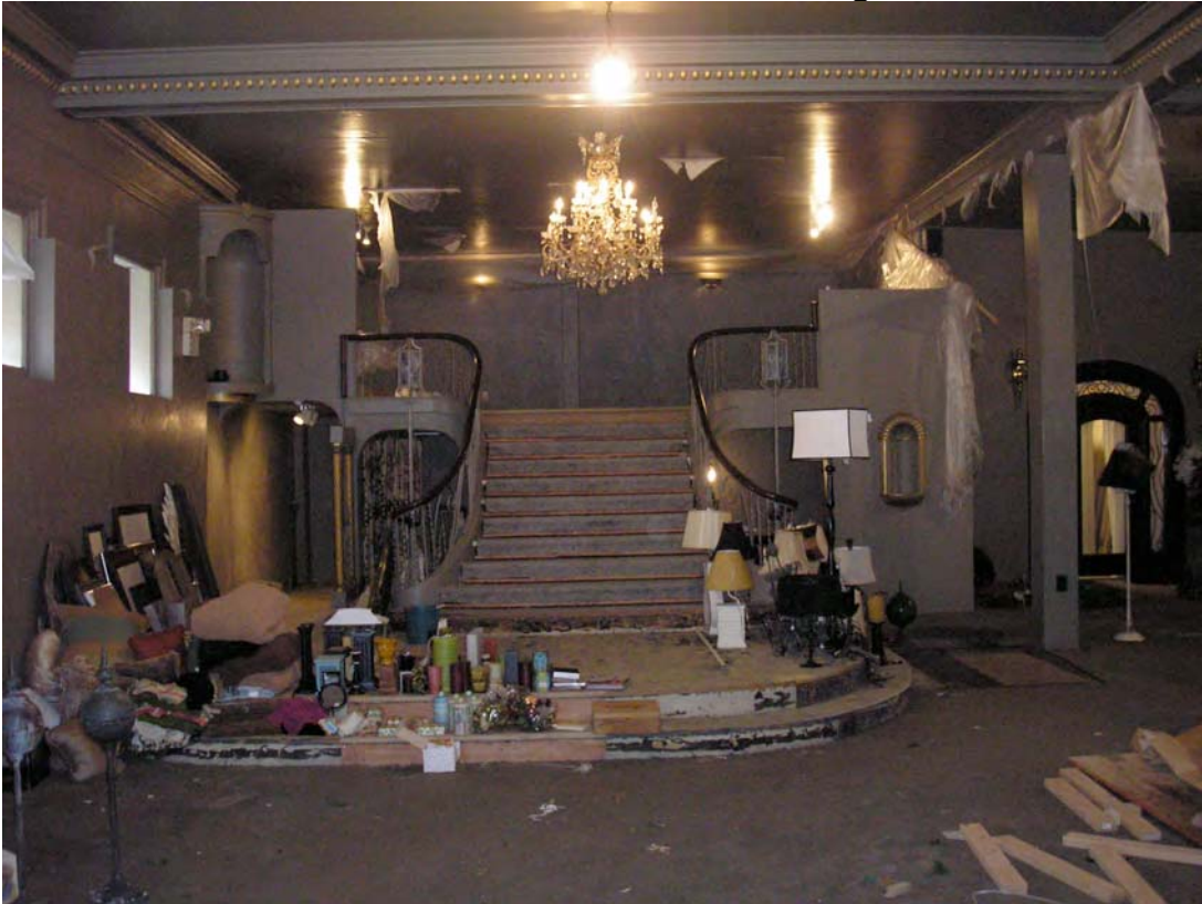
Level 1 Mezzanine Stairs & Interior Ceiling Beam Detail
