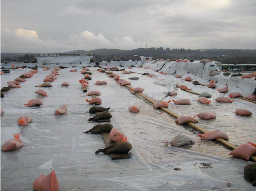
Second Temporary Roof In Place
